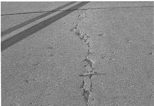
Figure E-3. Severity Crack.
