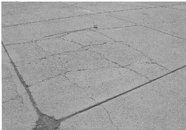
Figure E-12. Intersecting Cracks.
