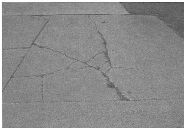
Figure C-3. Divided Slab.
