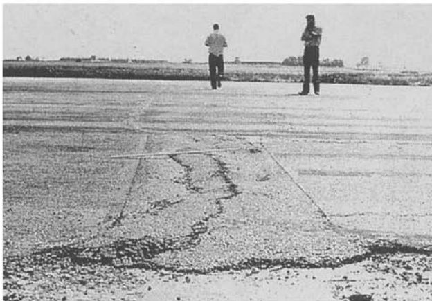
Figure D-10. Patching and Utility Cut Patch.
