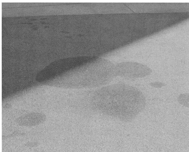
Figure D-9. Oil Spillage.
