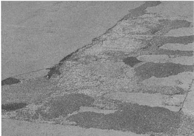
Figure C-16. Scaling, Map Cracking, and Crazing.
