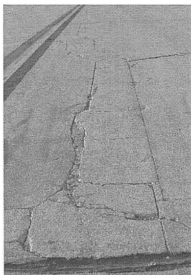
Figure E-7. Patching, Large.
