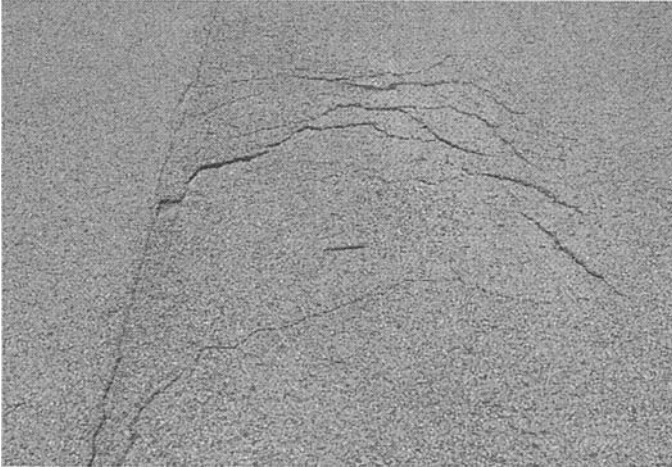
Figure D-15. Slippage Cracking.
