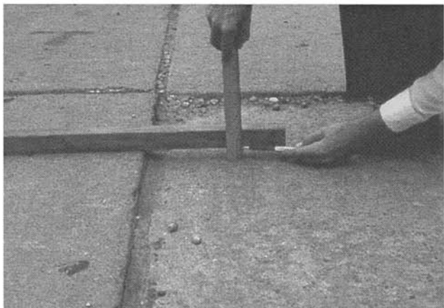
Figure C-5. Faulting.
