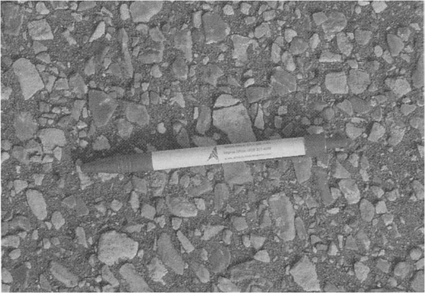
Figure D-11. Polished Aggregate.
