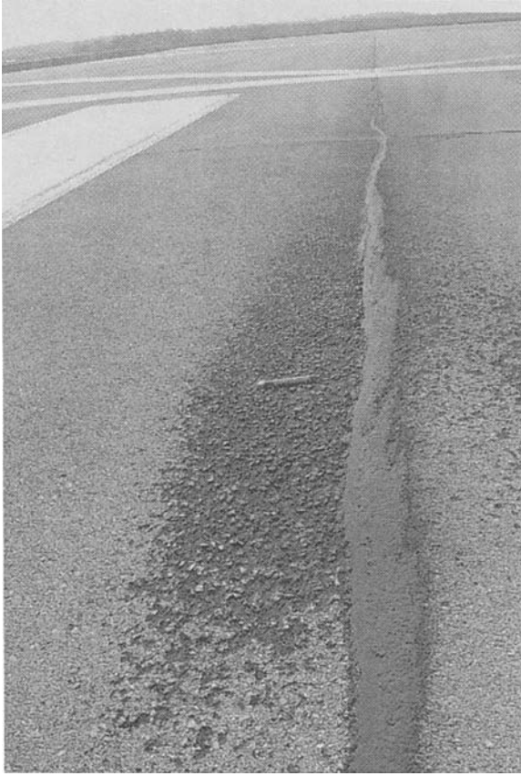
Figure D-6. Jet Blast Erosion.
