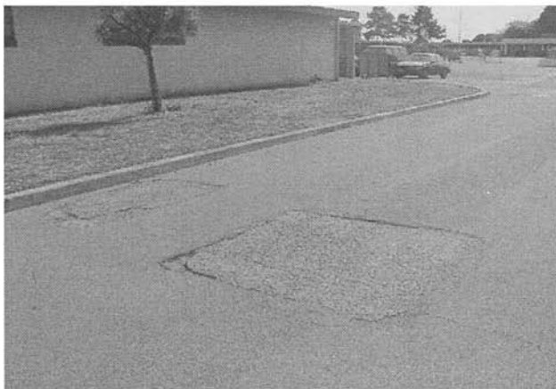
Figure B-11. Patching and Utility Cut Patching.
