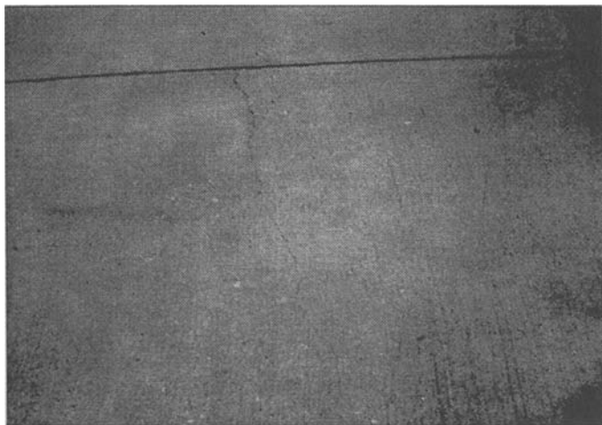
Figure C-17. Shrinkage Cracks.
