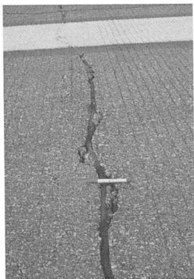
Figure D-8a. Longitudinal and Transverse Cracking.
