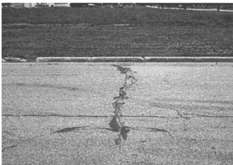
Figure B-10. Longitudinal and Transverse Cracking.
