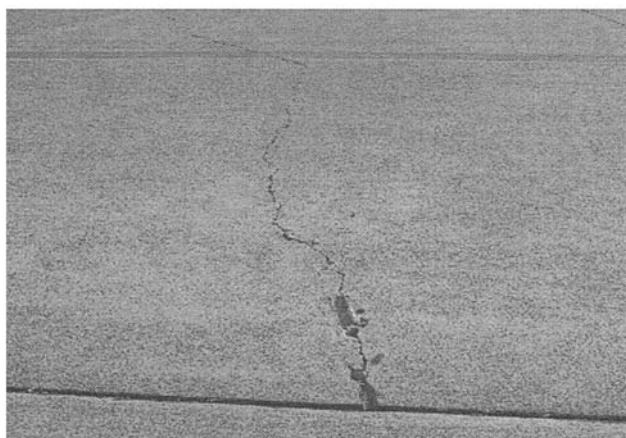
Figure E-3. Longitudinal Crack.
