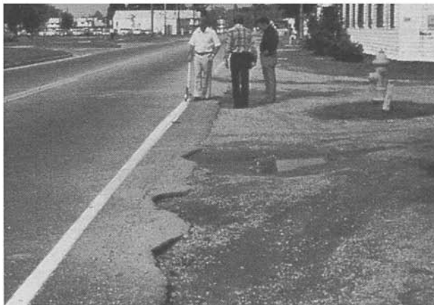
Figure B-7. Edge Cracking.
