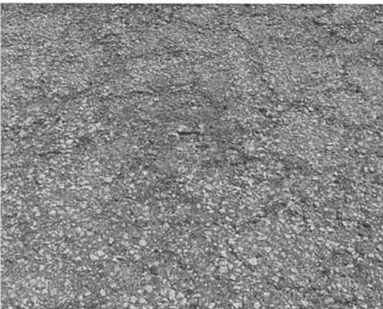
Figure D-12a. Raveling and Weathering.
